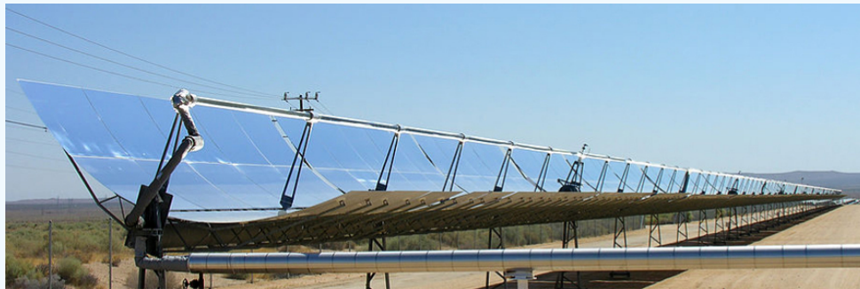
Figure 2.3.7: Parabolic trough collectors are used to generate electricity in southern California. (credit: “kjkolb”/Wikimedia Commons)
