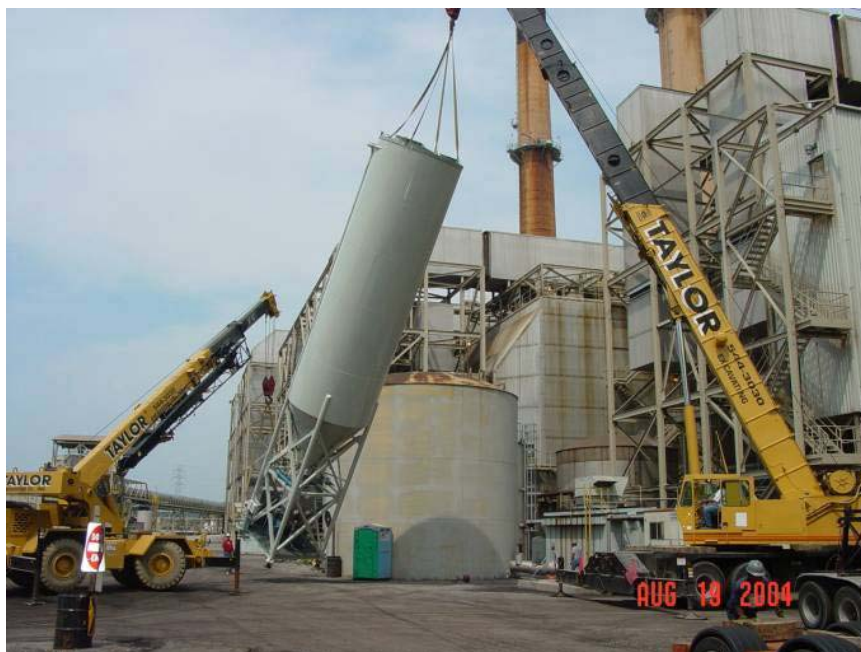
Figure 4. Photo of Injection Silo Installation at Meramec.
