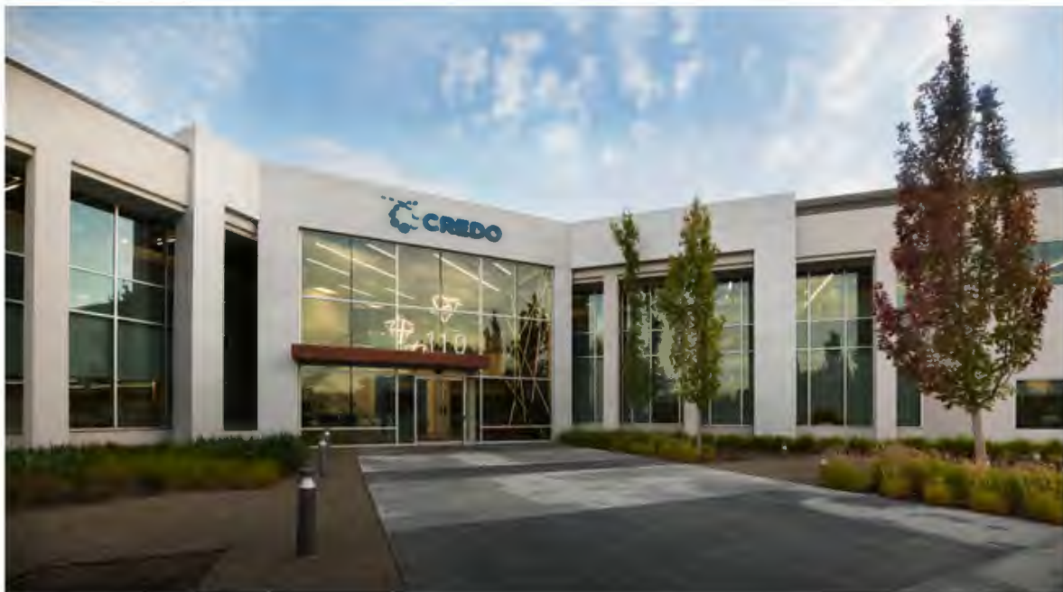
Credo Facility at 110 Rio Robles
