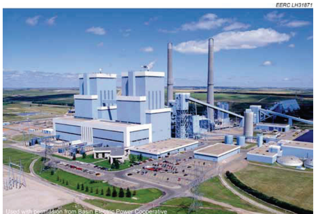
Figure 1 – Antelope Valley Station, near Beulah, North Dakota.
