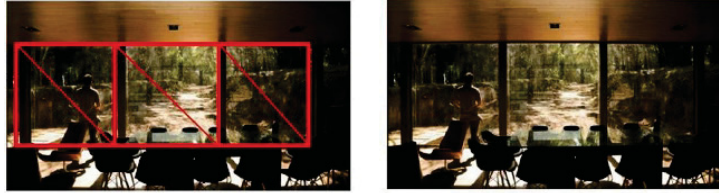
Figure 25 : Comparative structures. With diagonals (Pratt), without them (Vierendeel). Pabellón. (Source: Ferrer & Alarcia, 2014)
