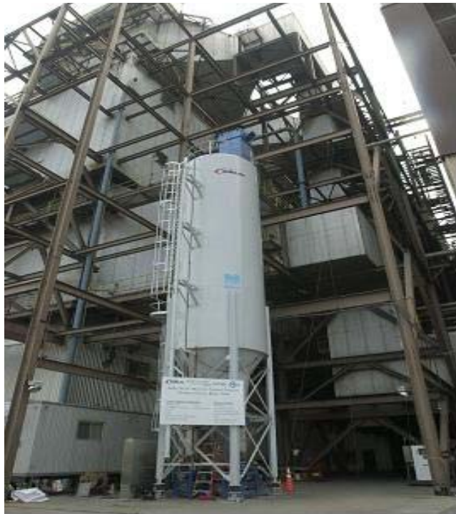
Fig 1. Carbon Injection Storage Silo and Feeder Trains Installed at PPPP.
